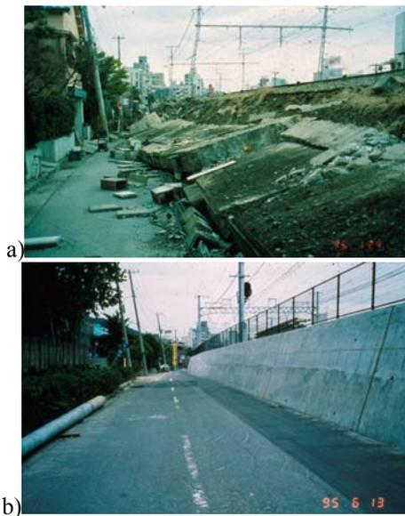
Fig. 13 a) Collapse of a gravity type (leaning type) RW during the 1995 Kobe Earthquake; and b) reconstructed GRS-RW having a stage-constructed FHR facing (Tatsuoka et al., 1996, 1997a & b)
