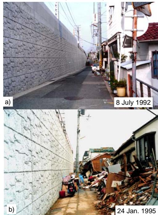
Fig. 12. A GRS RW having a FHR facing at Tanata, Japan: a) immediately after wall completion; and b) immediately after the 1995 Kobe Earthquake (Tatsuoka et al., 1996, 1997a & b)
