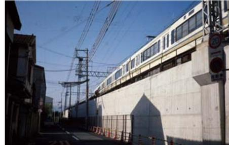
Fig. 3. Amagasaki wall in Hyogo Prefecture: the first large scale GRS RW supporting directly tracks for a very busy rapid railway (JR Kobe line), constructed during 1991-1992 under a severe space restriction; average wall height= 5 m & total length= 1,300 m.
