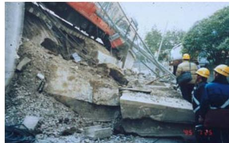
Fig. 11. Gravity type RW without a pile foundation at Ishiyagawa that collapsed during the 1995 Kobe Earthquake (Tatsuoka et al., 1996, 1997a & b)
